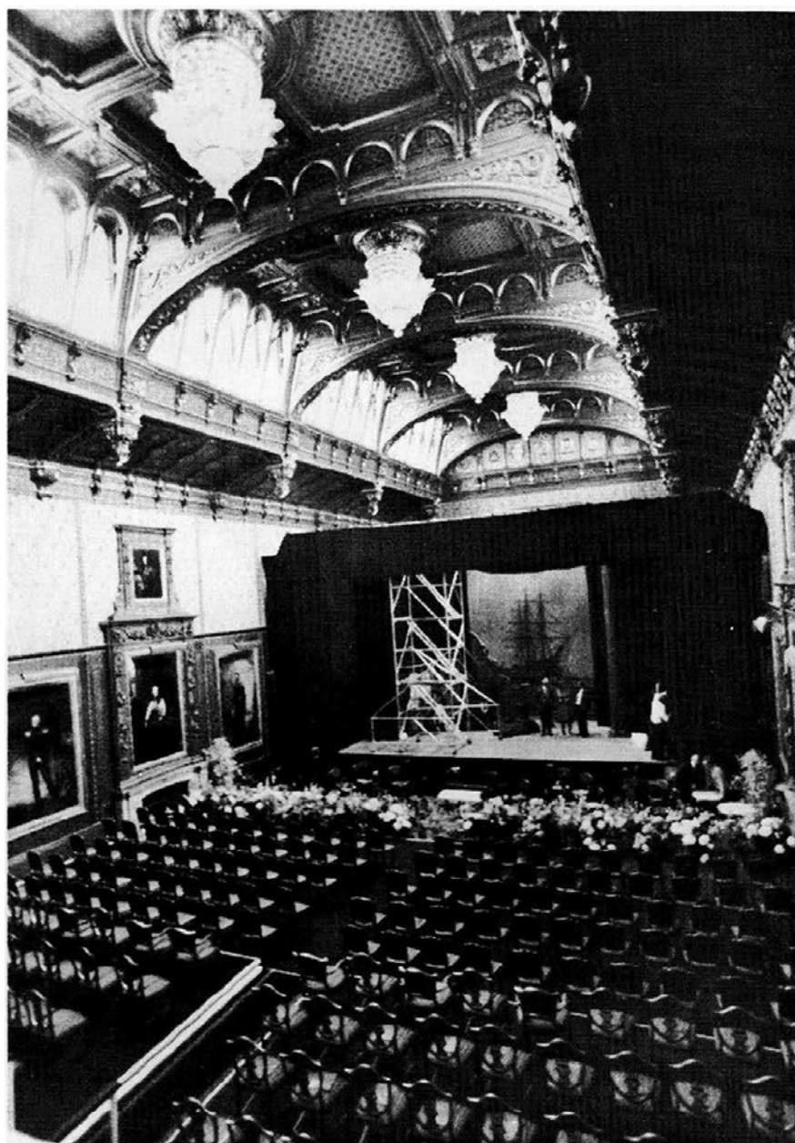
The Waterloo Chamber during the erection of the proscenium arch.
